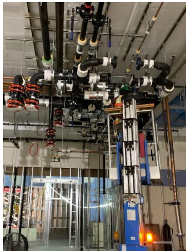
04/22/24 – Installed piping above Level G Mechanical Room 1130
