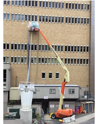
04/29/24 – OHS C-Wing Brick Demo/Abatement
