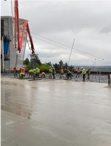
04/29/24 – Concrete placing at level 4 vegetated roof
