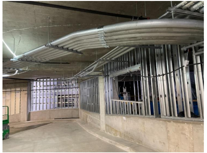
04/26/24 – Infill framing and conduit sweeps at NW corner of P3
