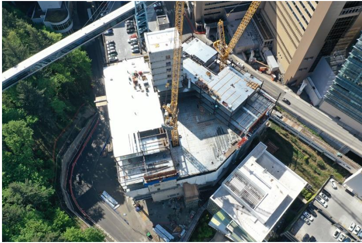
04/23/24 – Drone view of jobsite
