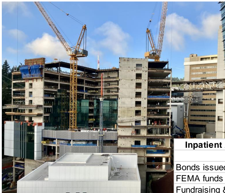
Construction as of 9/13/24
