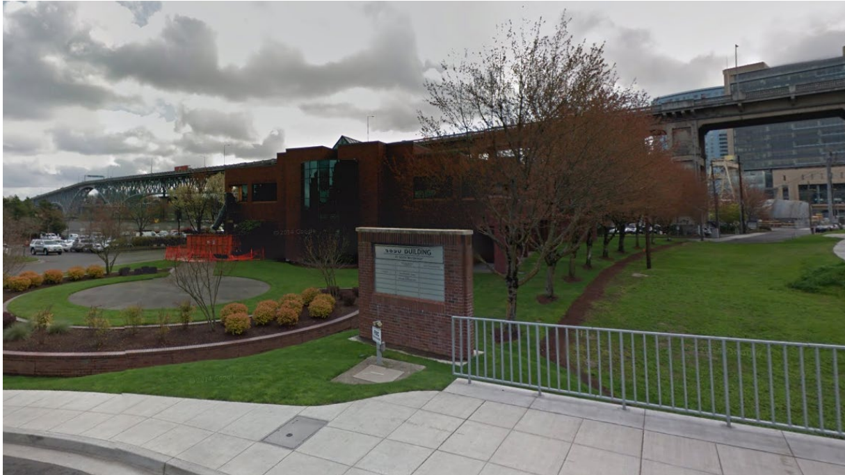
3030 SW Moody Building – gathering place for On Campus Emergencies
