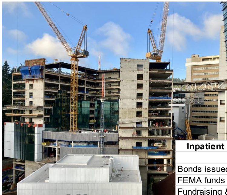
Construction as of 9/13/24
